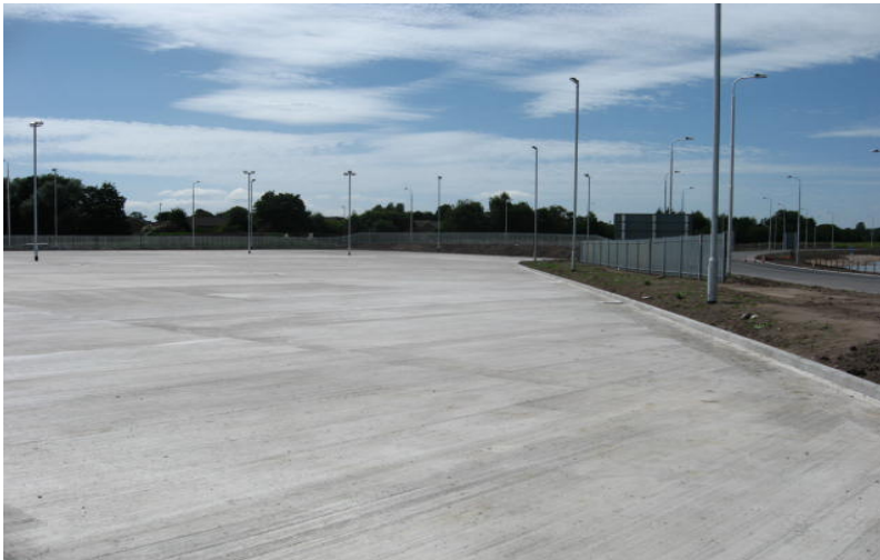
VOSA site - concrete slabs
