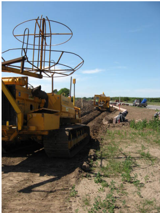
Land drainage installation near Rakes Lane
