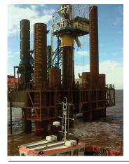
To build the quay wall, 40m long steel piles will be driven into the sea bed using a range of piling techniques (the picture to the left shows the first of the piles in position in the gate).
